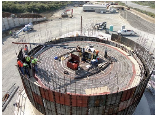
A view of the work deck and internal scaffolding reveals the Jump-O-Form process in construction of a 45' diameter fly ash silo at the AEP Mitchell Power Station, Moundsville, WV.
